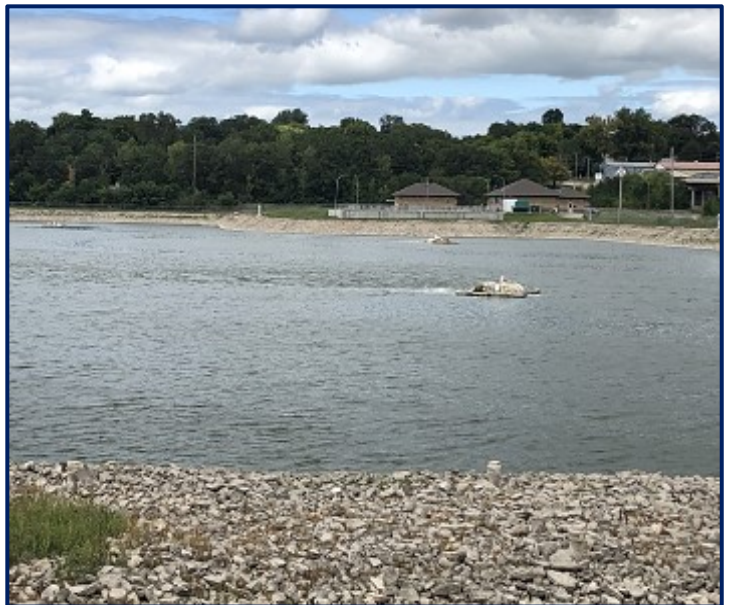
Lagoon with three surface aerators – not meeting oxygen or mixing requirements
