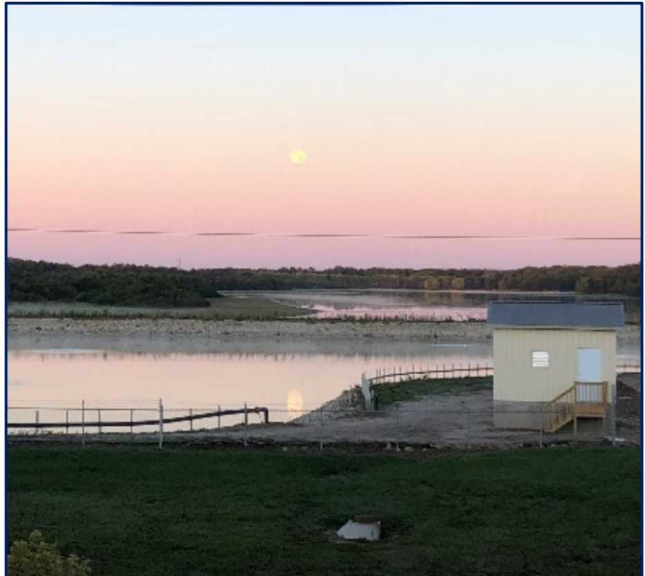
Blower building at Spring Valley Lagoon
