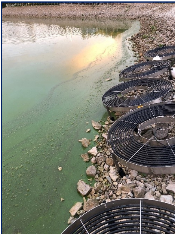
Disks along shore during ADS system installation
