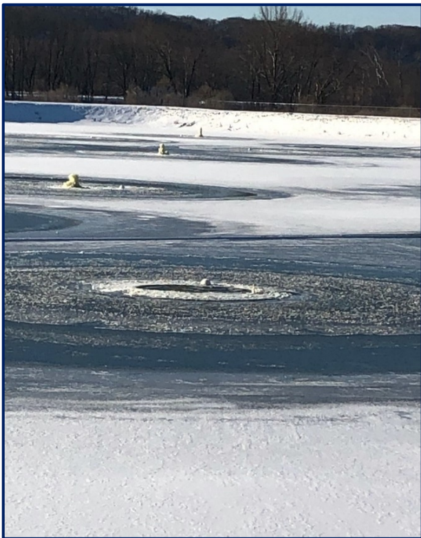
Winter operation with open water above the diffusers and stalagmite growth
