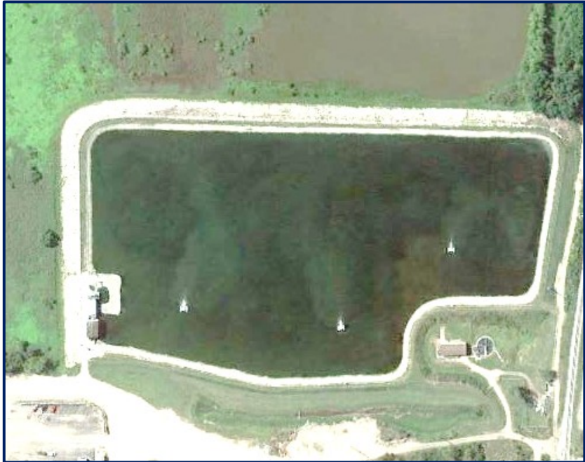
Aerial view of lagoon with surface aerators before ADS fine bubble treatment
