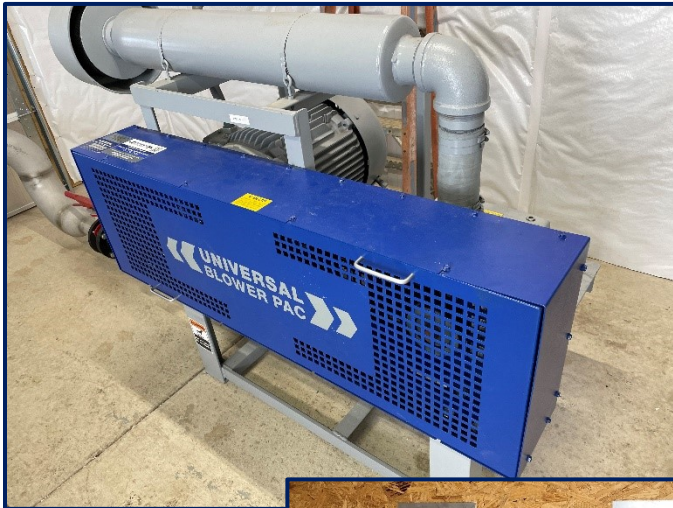
Blower with Variable Frequency Drive Control Panels
