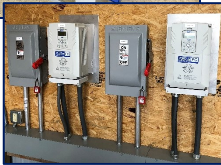
Blower with Variable Frequency Drive Control Panels
