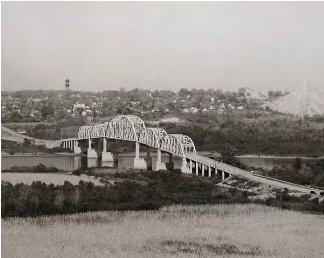
Historic photo of Spring Valley featuring the original bridge built in 1934. Photo by Art Kistler, IDOT.
